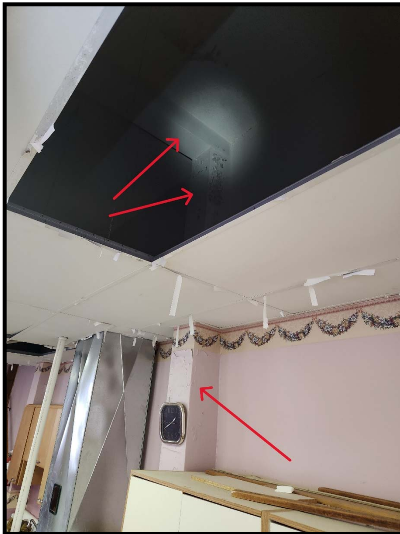
Photograph 10: location of finished steel columns and beams in newer addition
