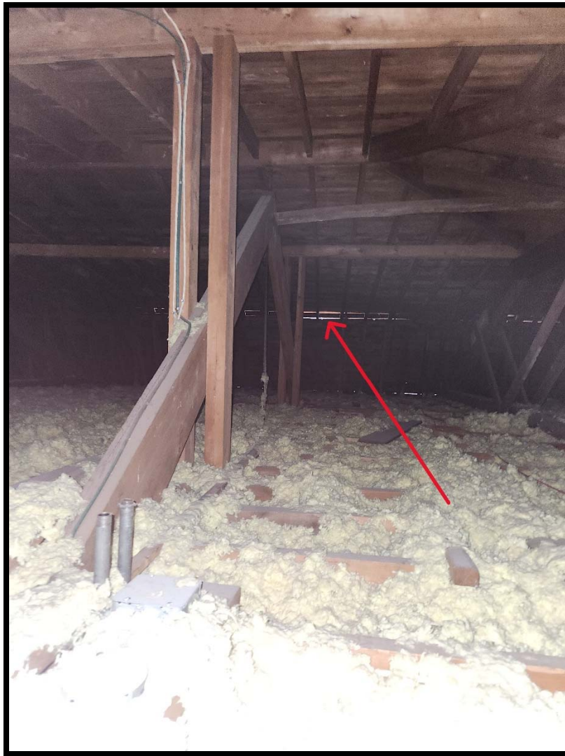
Photograph 14: typical roof truss, purlins and rafters; daylight showing
