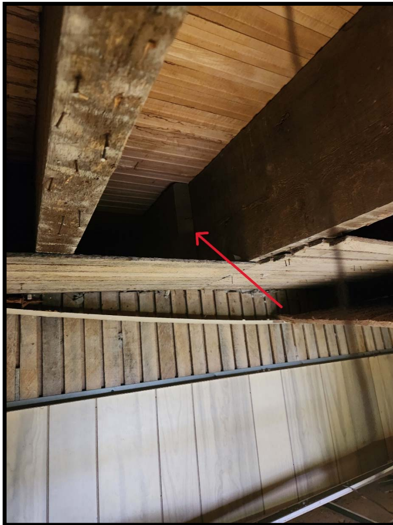
Photograph 8: joists spliced atop of load bearing wall
