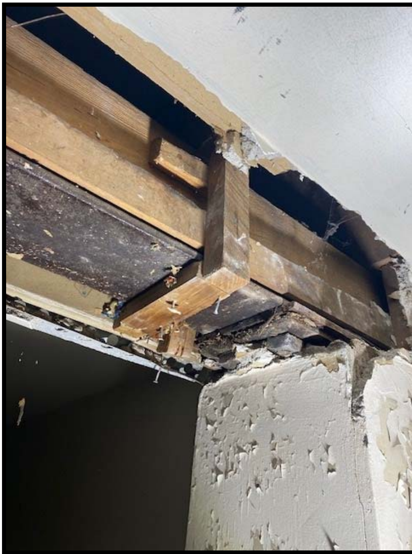
Photograph 12: steel beam atop of column in newer addition
