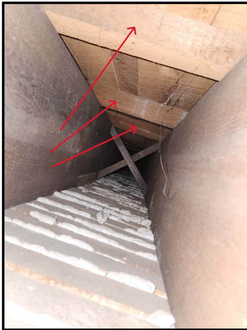
Photograph 9: shims for sloped floor
