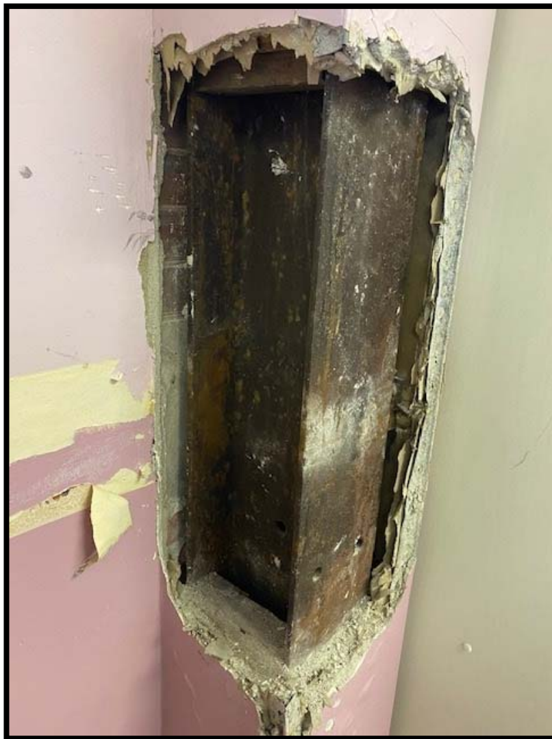
Photograph 11: steel column in newer addition
