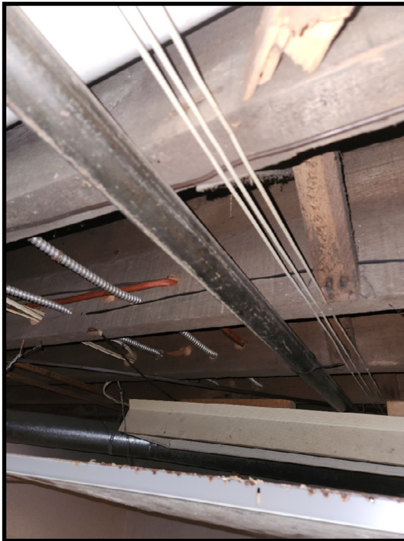
Photograph 6: general condition of joists over basement
