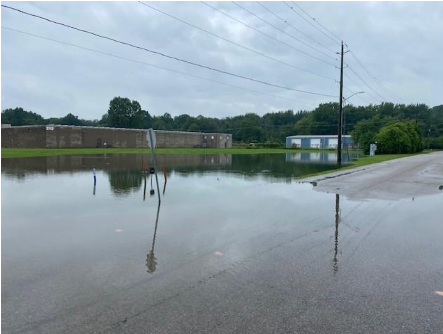
Image 7: Roadway flooding at corner of Finney Street and Gilbert Street on July 29, 2023
