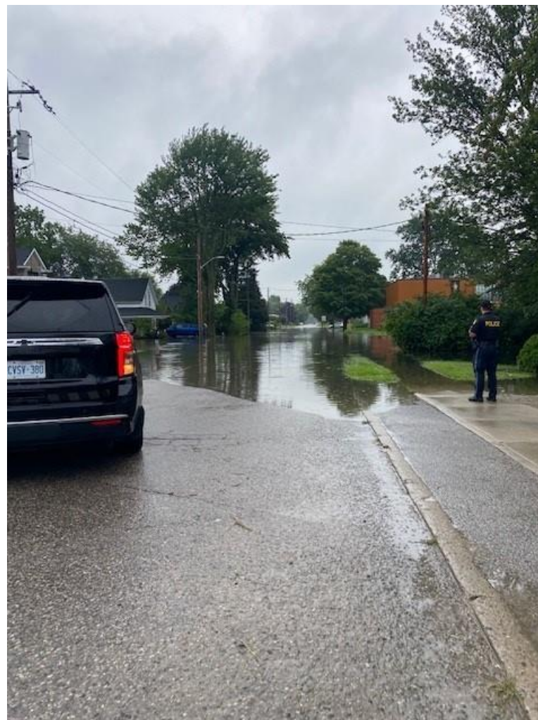
Image 2: Roadway flooding adjacent to St. Mary's Roman Catholic Church on July 29, 2023
