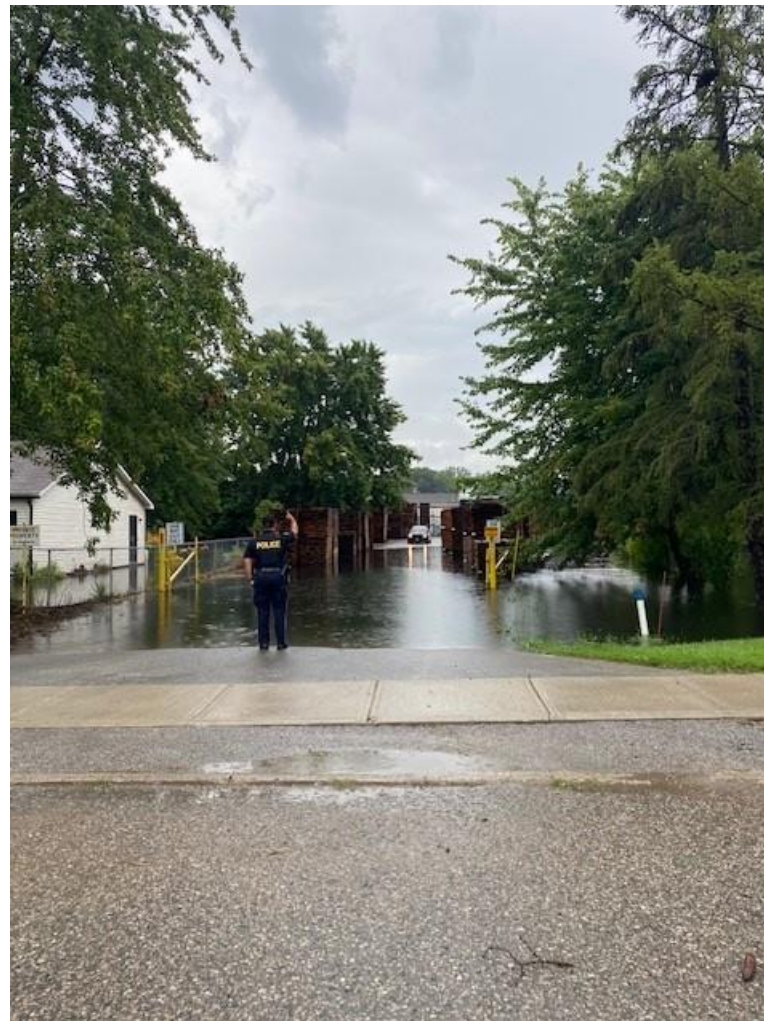
Image 6: Roadway flooding at 167 Pioneer Line on July 29, 2023 Existing Storm Sewer Diameter: 150mm Proposed Storm Sewer Diameter: 450mm
