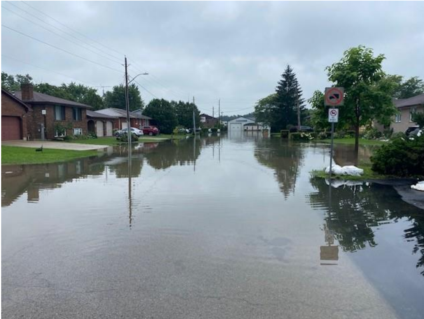
Image 9: Roadway flooding on Anne Street looking towards Finney Street on July 29, 2023 Existing Storm Sewer Diameter: 300mm Proposed Storm Sewer Diameters: 450mm and 525mm
