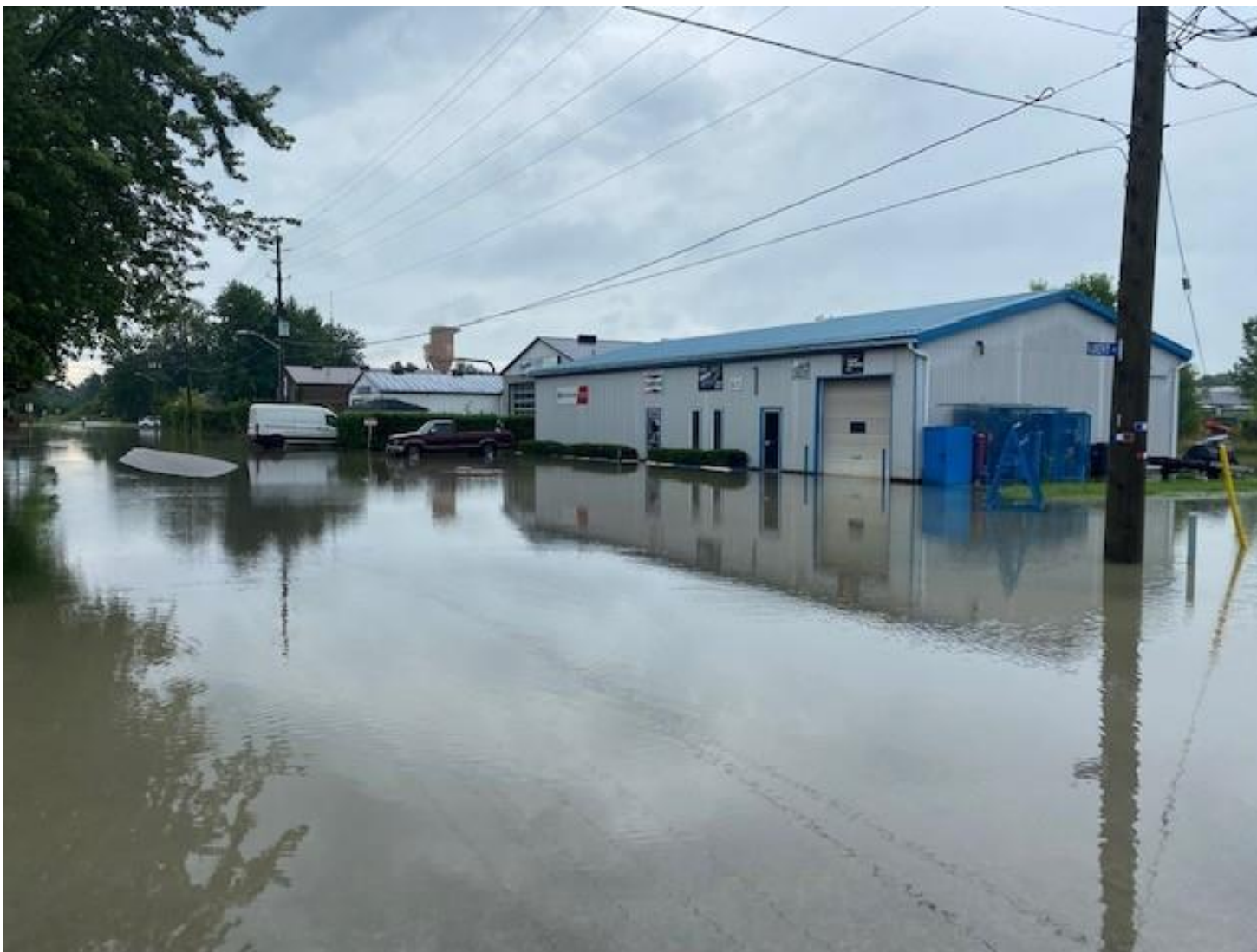
Image 8: Roadway flooding at the corner of Finney Street and Gilbert Street on July 29, 2023 Existing Storm Sewer Diameter: 300mm Proposed Storm Sewer Diameters: 525mm and 600mm
