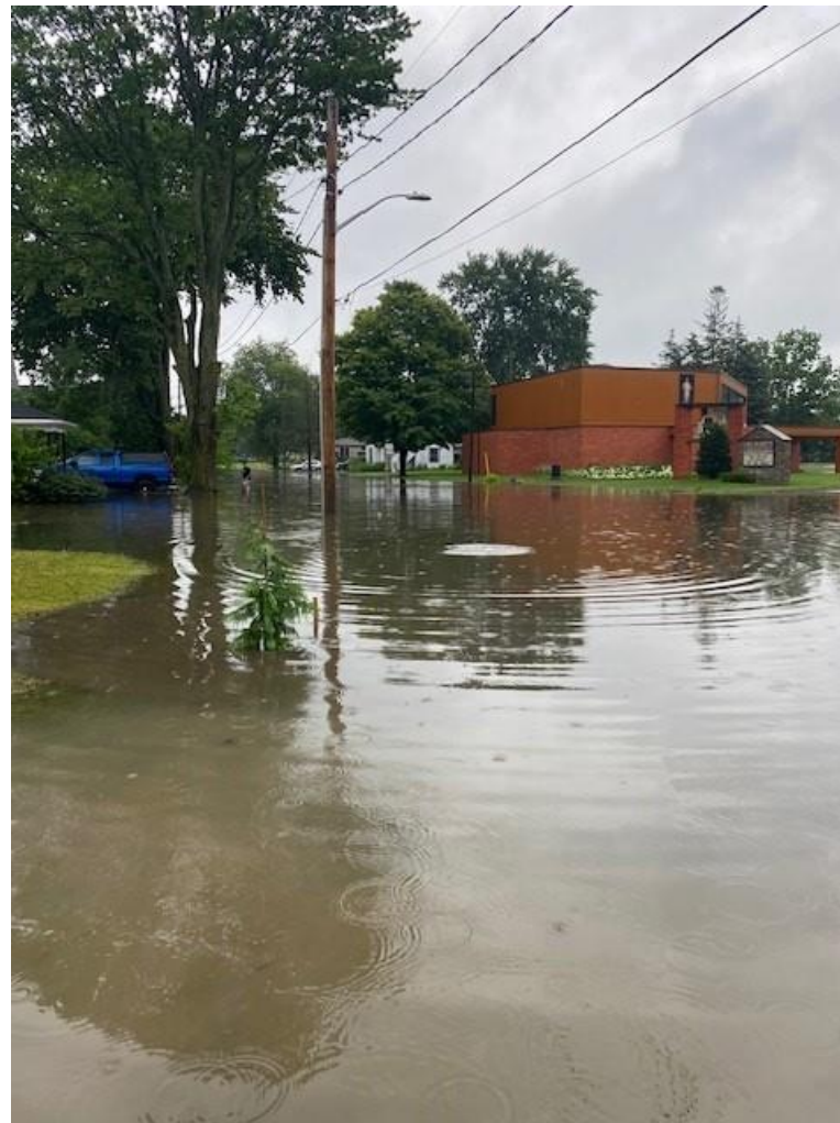
Image 4: Roadway flooding at St. Mary's Roman Catholic Church on July 29, 2023
