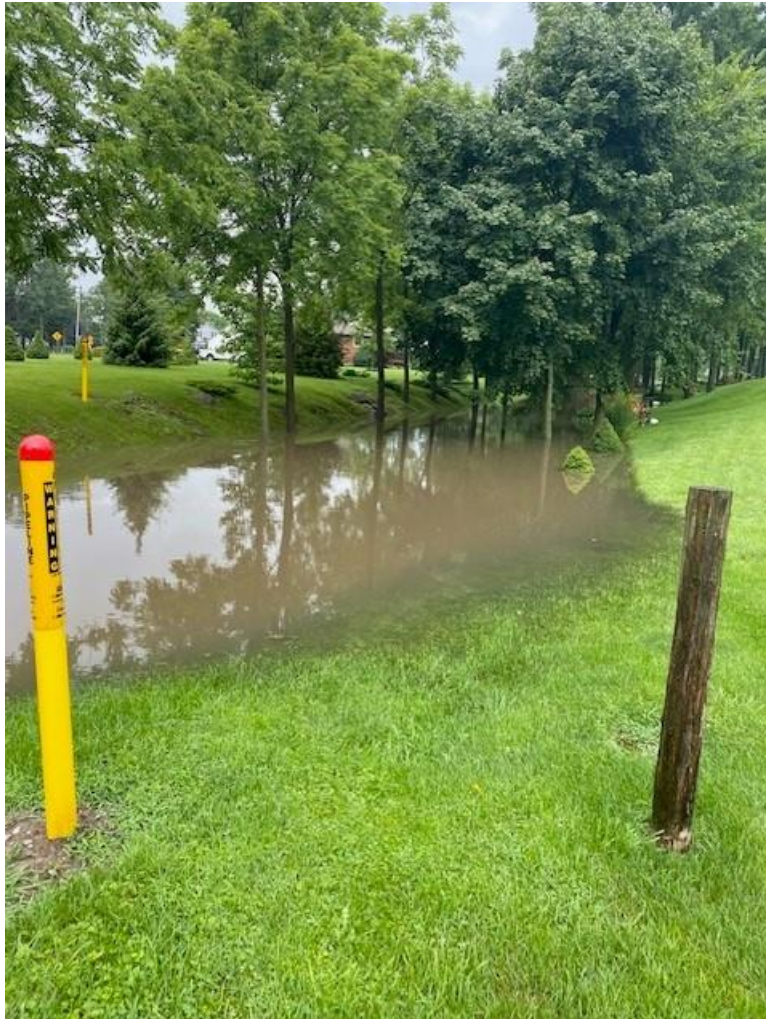
Image 10: Flooding within swale adjacent to 10990 Graham Road on July 29, 2023
