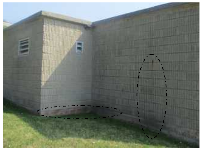
Moisture staining and damaged on the north elevation of Building C.
