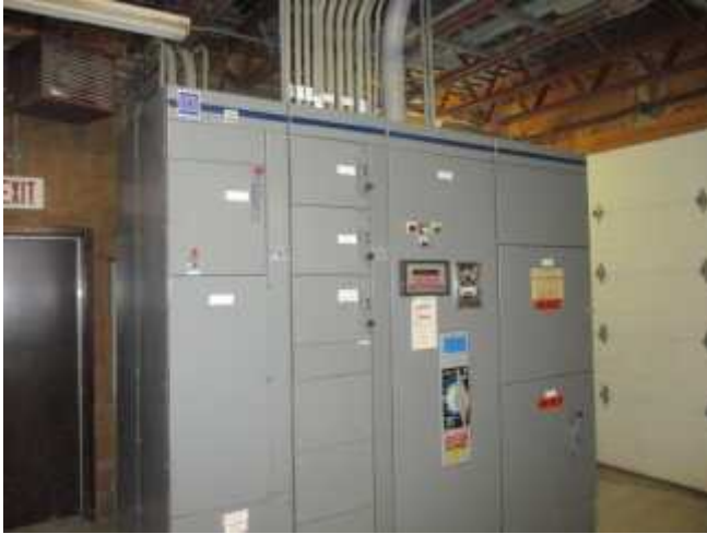
Main electrical distribution and disconnect switch serving all buildings.
