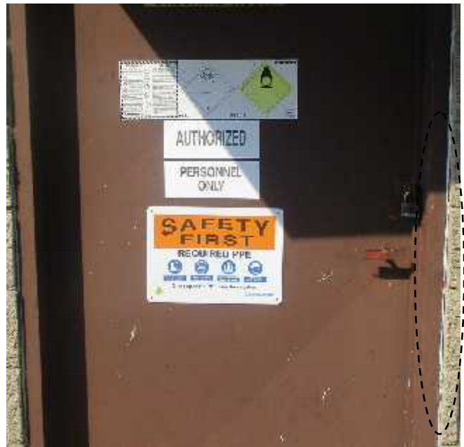
Deteriorated sealants at the door perimeter of Building C.
