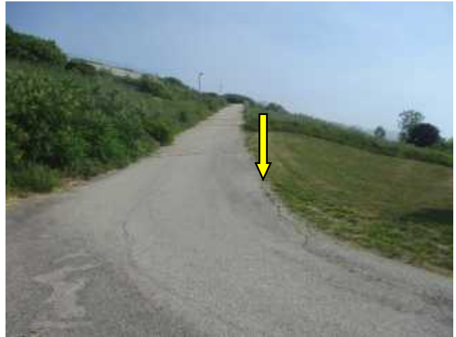
General view of asphalt pavement roadway at the central portion of the site. Areas of longitudinal cracks noted.
