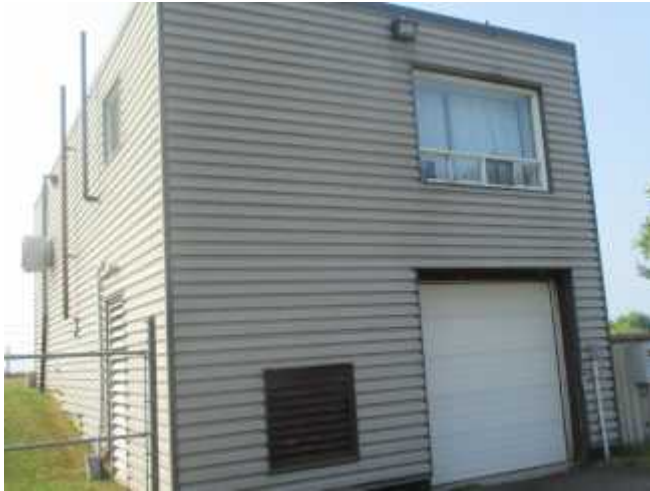
View of prefinished metal siding on north (right) and west (left) elevations of Building A.
