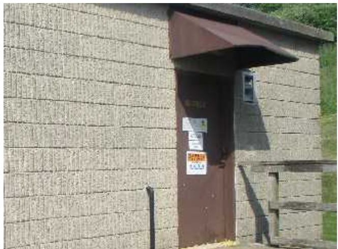
Corrosion was noted on the main entrance door and door hardware of Building C.
