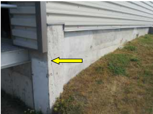
Minor cracking was noted on the foundation wall.
