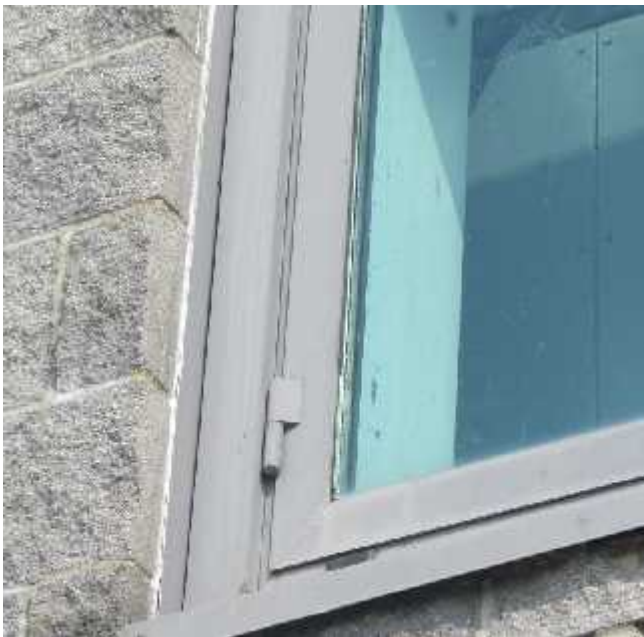
Split sealants around the windows of Building B.
