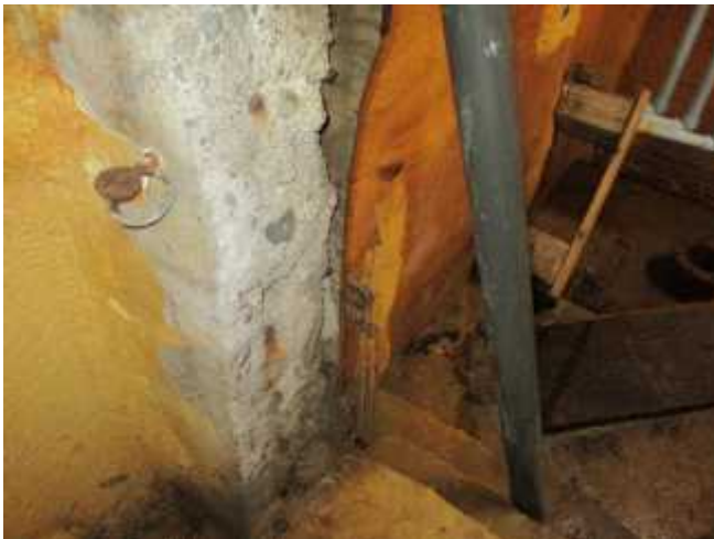
Water infiltration was noted within the basement of Building C.
