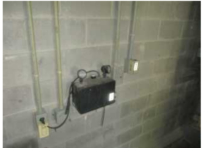
Typical emergency light and battery pack located within Building A.
