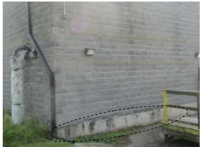
Cracks and staining on the exterior face of the west wall of Building B.
