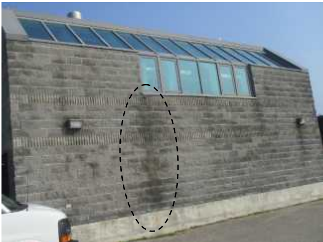
Moisture stained walls on the south elevation of Building B.
