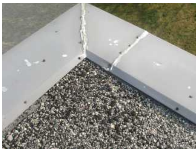
Hardened and deteriorated sealants were noted on the joints of parapet flashing.
