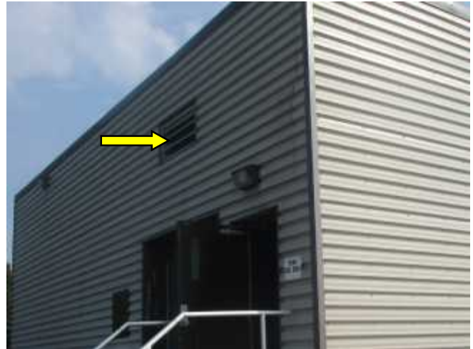
Ventilation louvre on the west elevation of Building A.
