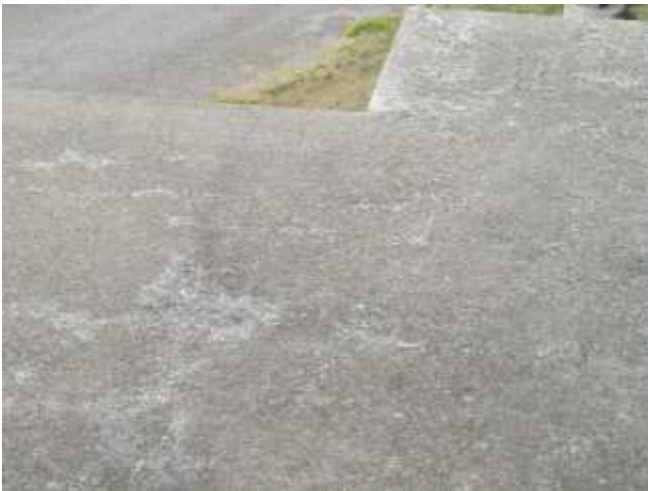
Surface pitting noted on the exposed roof concrete.
