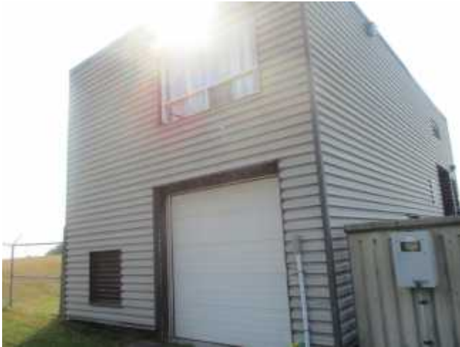
Prefinished metal roll-up door on the north elevation of Building A.
