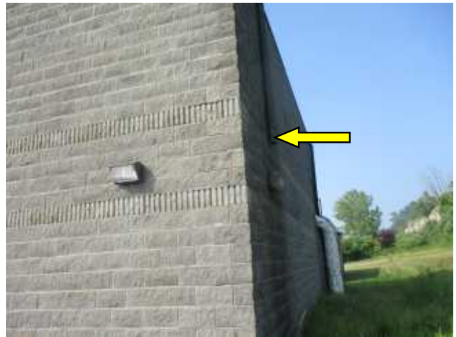
Missing piece of a downpipe on the north elevation of Building B.
