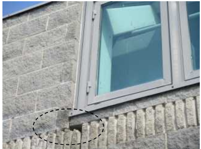
Missing mortar was noted below corner of the window.
