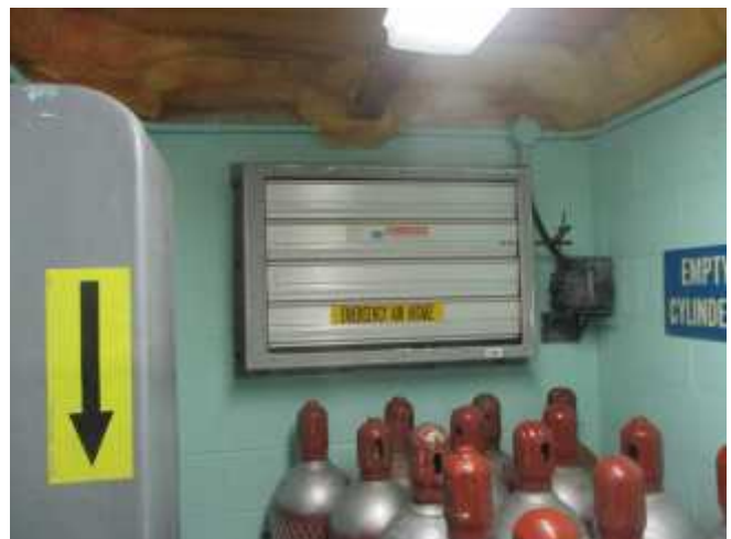
Interior view of emergency air intake unit in Building C.
