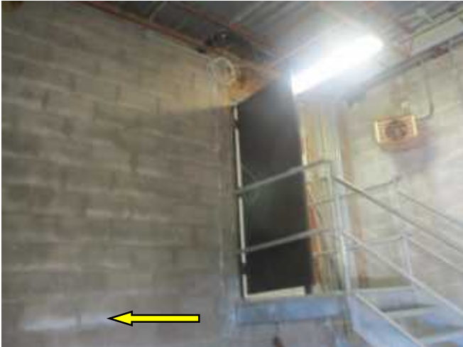
Moisture staining and efflorescence were noted on the interior walls of Building A.
