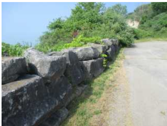
Shifted and leaning units were noted on the south wall.
