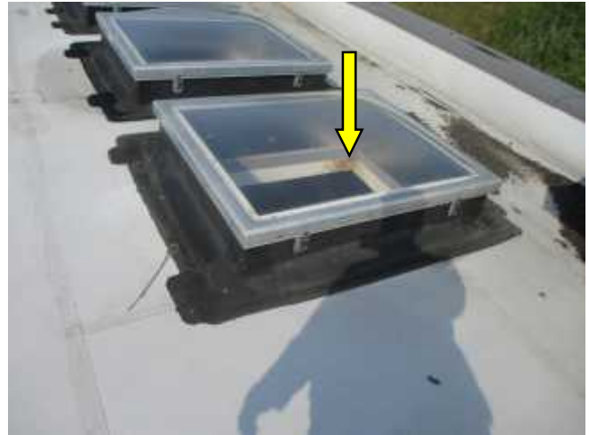
Moisture staining on the inner side of the skylight opening indicates leakage, likely caused by failure of perimeter sealant.
