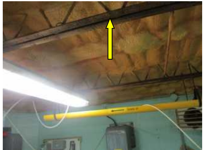
Heavy corrosion noted on the open web steel joist systems supporting the roof decking.
