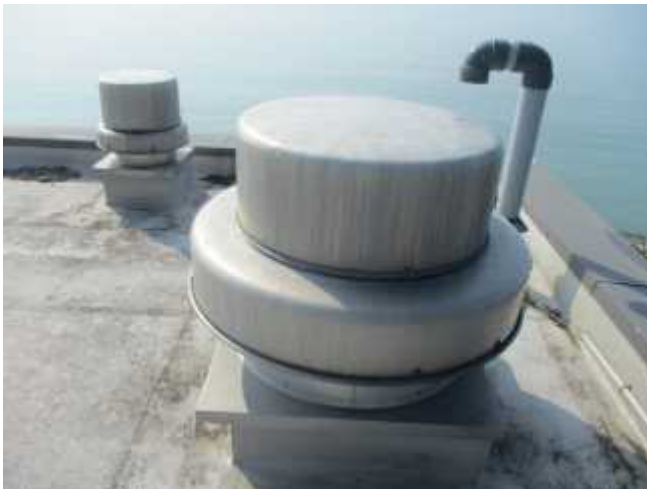
Rooftop hooded ventilation units atop Building B.
