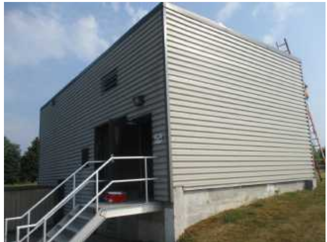
Prefinished metal siding on the south elevation was noted to be in good condition.
