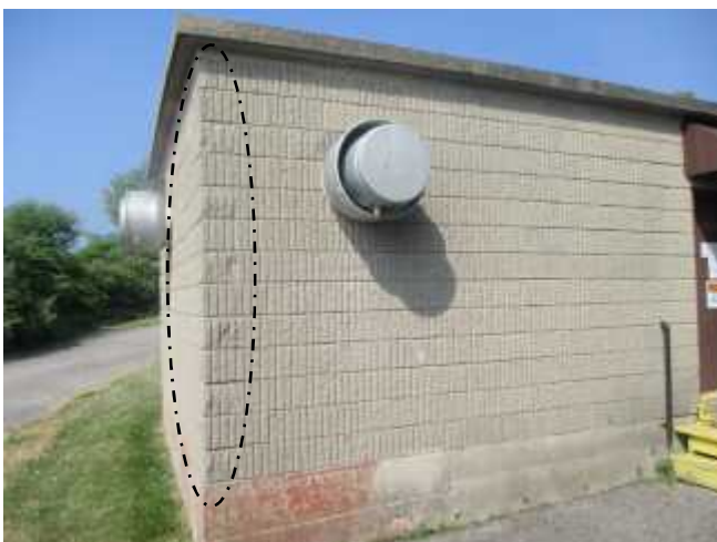
Spalled concrete blocks on the southeast corner of Building C.
