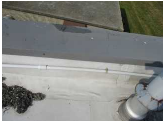
Wrinkled and tented membrane noted along the roof edge.
