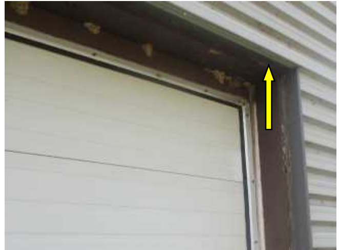
Deteriorated sealants at perimeter of a garage door of Building A.
