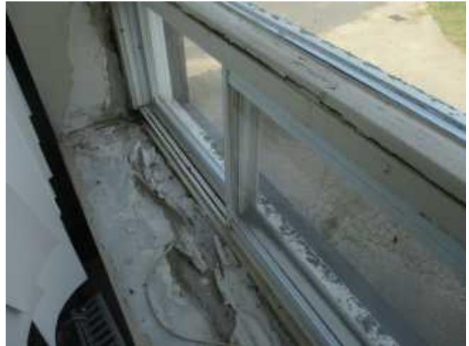
Evidence of heavy leak and mould growth on the window frame was noted on the north face of Building A.
