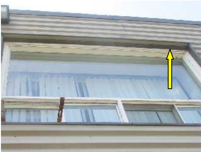
Window perimeter sealants were noted to be in poor condition in Building A.
