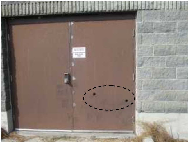
Unsealed holes on the secondary entrance door of Building B.
