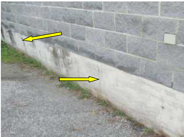
Surface cracks minor delamination and moisture staining were noted on the exterior face of foundation walls.
