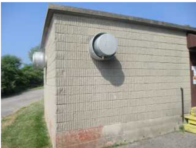
Wall-mounted hooded ventilation units serving Building C.
