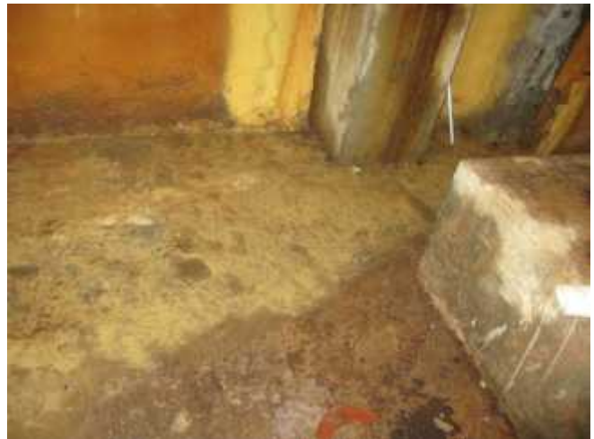
Surface deterioration was noted at the basement floor slab.
