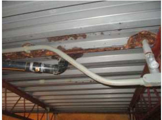
Corrosion was noted on the underside of the floor decking.
