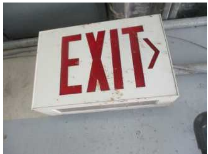
An exit sign with burnt-out light bulb in Building B.
