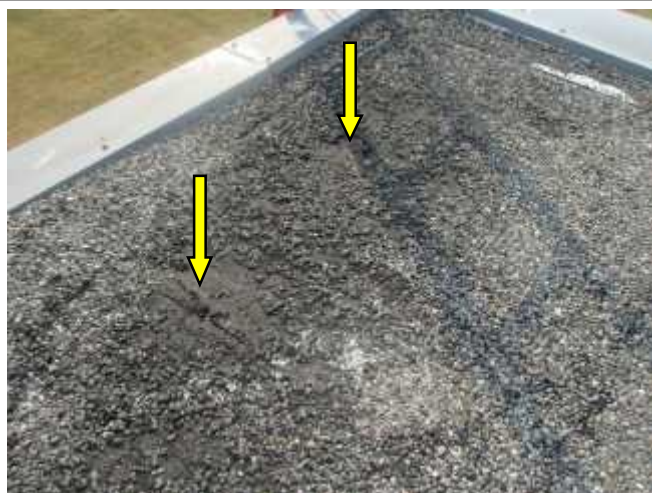
Exposed deteriorated membrane was noted on the southwest corner of the roof.
