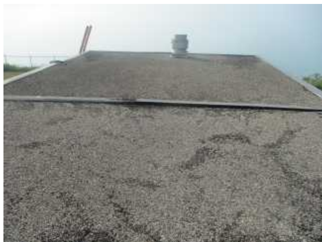
General view of the BUR system atop Building A.
