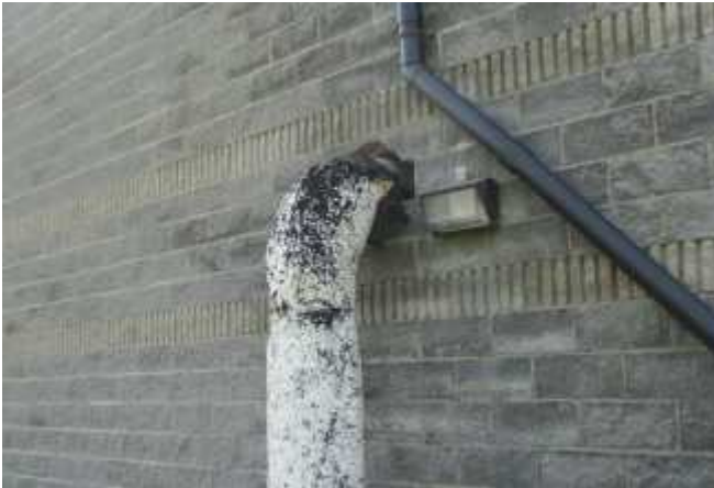
An unsealed pipe penetration on the exterior wall of Building B.
