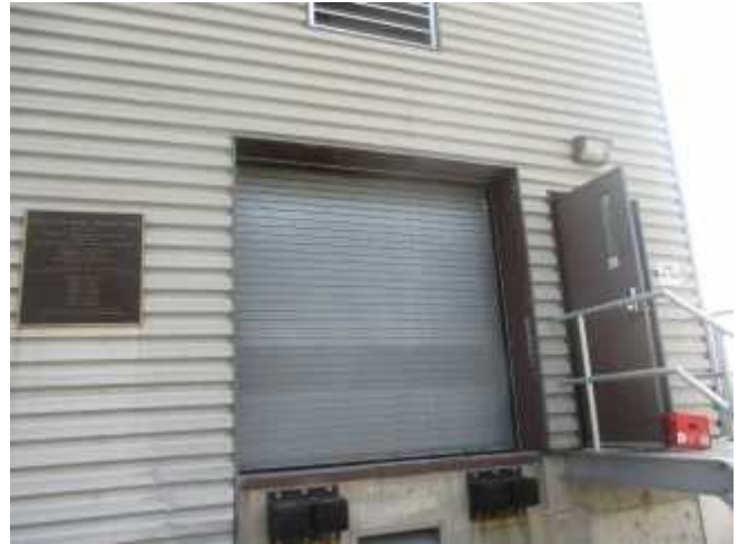
Metal roll-up door serving a loading dock on the west elevation of Building A.
