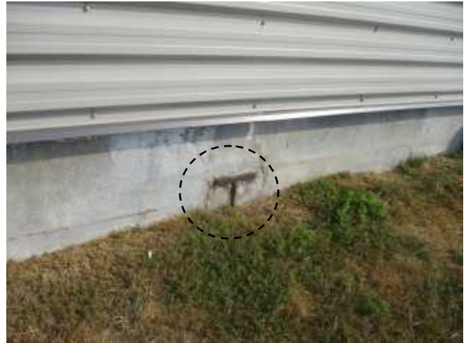
Exposed corroded steel was noted imbedded at the foundation wall of Building A. Epoxy coating may be considered.
