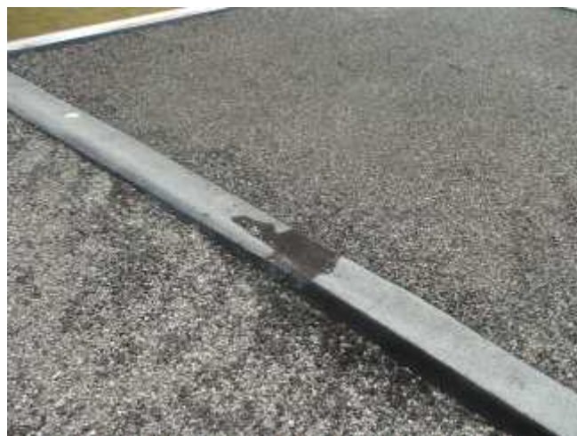
Modified bitumen roof membrane on the control joint of Building A
