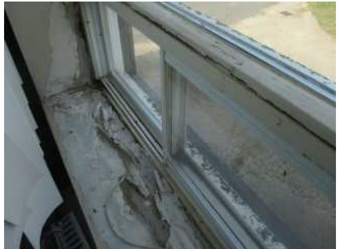
Moisture damage on the window sill on the north portion.
