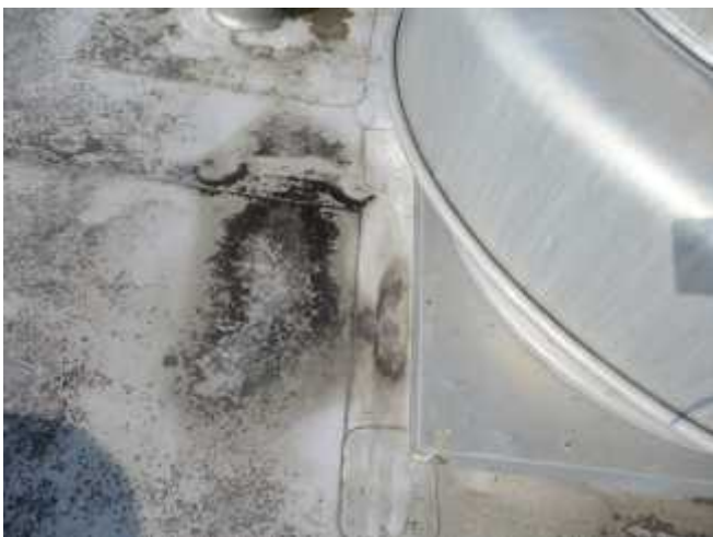
Ponding water and deteriorated membrane atop the roof.
