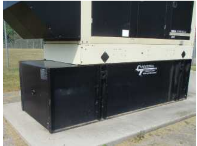
Generator storage tank.
