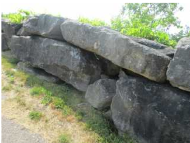
Evidence of minor erosion and shifted units observed at the south wall.
