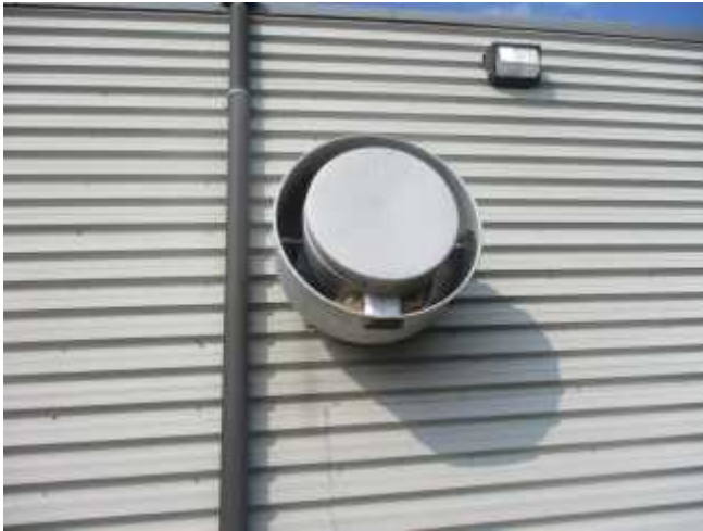
Hooded ventilation fan on the east elevation of Building A.
