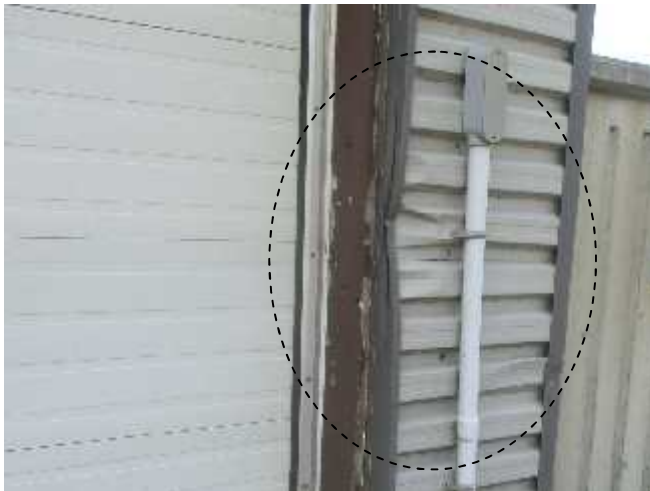
Damaged siding on the north elevation of Building A.
