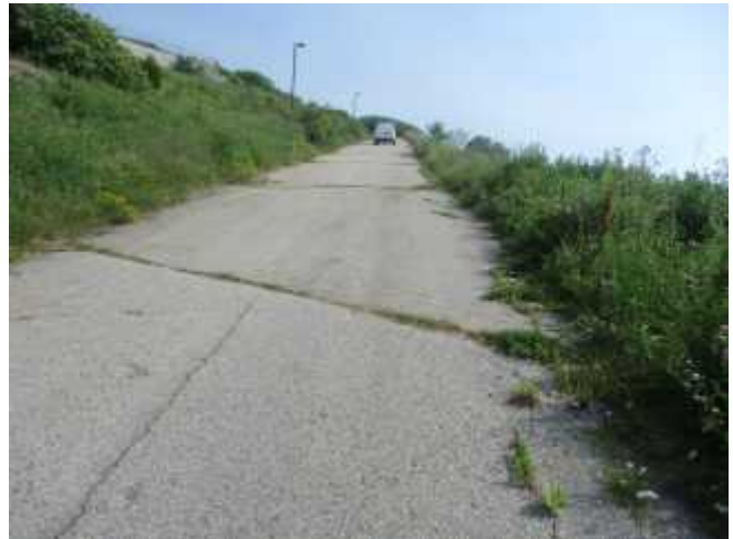
Cracking and growth within the cracks of the asphalt pavement.
