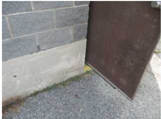
Fading and deteriorated finish on entrance of Building B.
