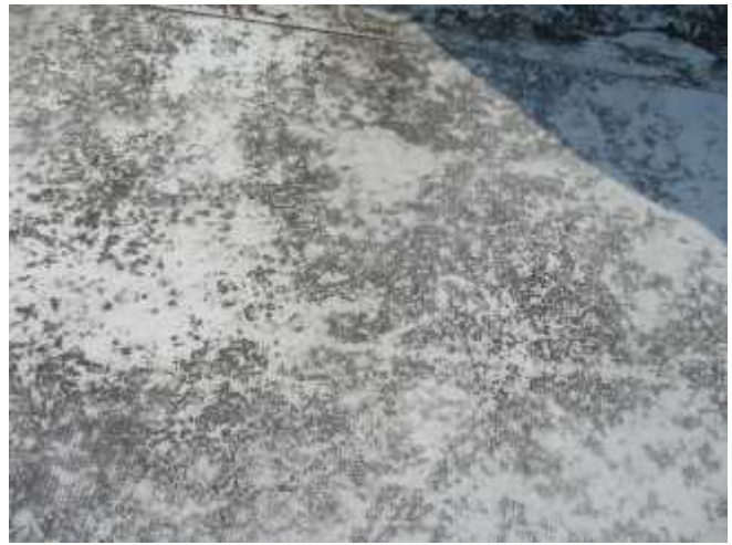
Deteriorated surface of the PVC membrane.
