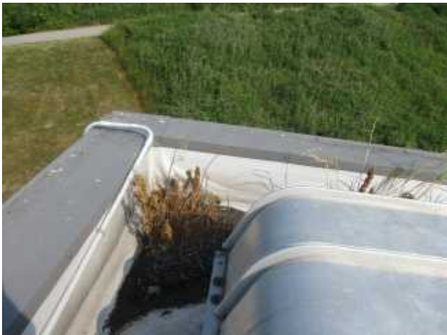
Debris accumulation and growth on the roof.
