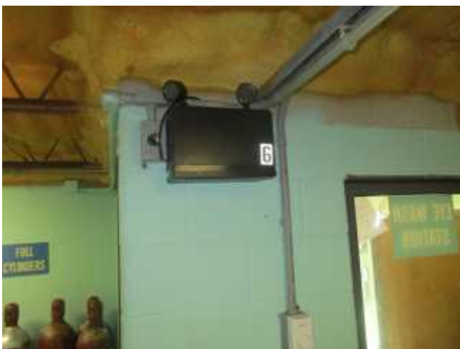
Typical emergency light and battery pack located within Building B.
