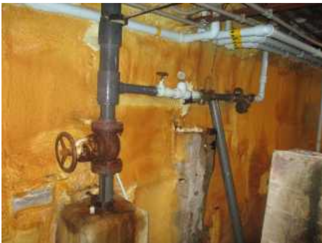
Corroding piping and valves noted in the basement of Building C.
