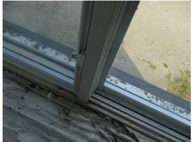
Mould growth is evident on the exterior face of window frame.
