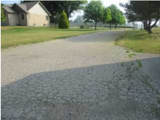
Asphalt pavement deterioration manifested in the form of severe alligator cracking on the north portion of the site.
