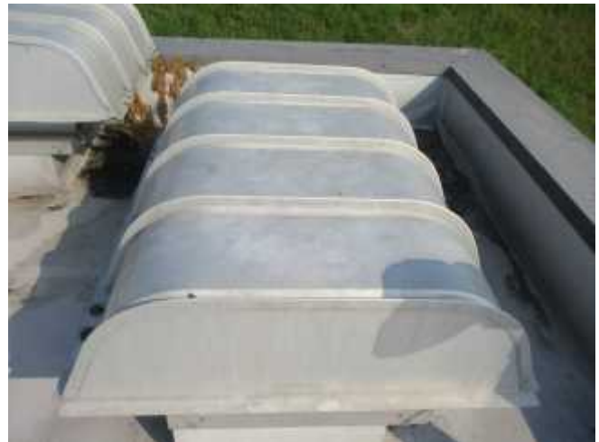
Air intake units on the roof of Building B
