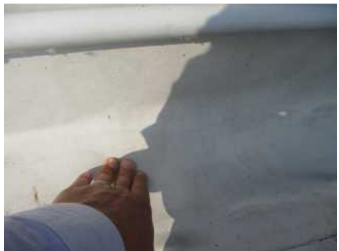
Tenting was noted to be severe along the west edge.
