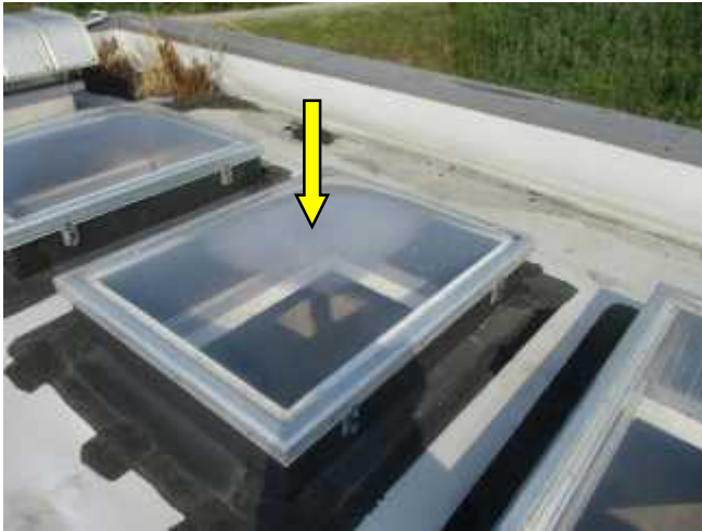
Presence of condensation between the panels of the skylight indicates failure of the hermetic seal.
