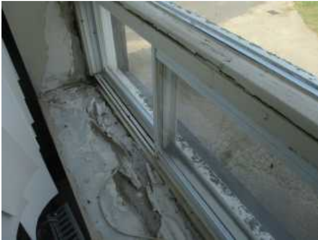
Damaged window sill of Building A where mould growth is suspected.
