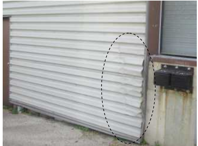
Impact damage on the cladding on the west elevation of Building A.
